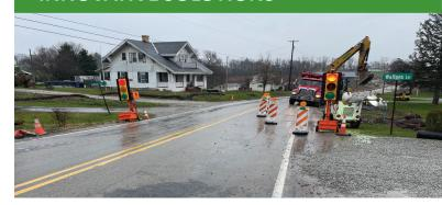
The construction team is using portable traffic signal systems throughout the project area. The smaller software-based system is ideal for short-term traffic control providing increased work-zone safety while maximizing traffic flow. Crews can focus on the task at hand instead of manually flagging traffic.
